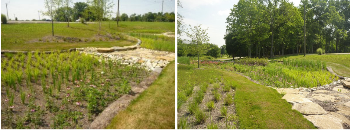
Figure 1214. Bioretention Basins (stormwater.wef.org)
