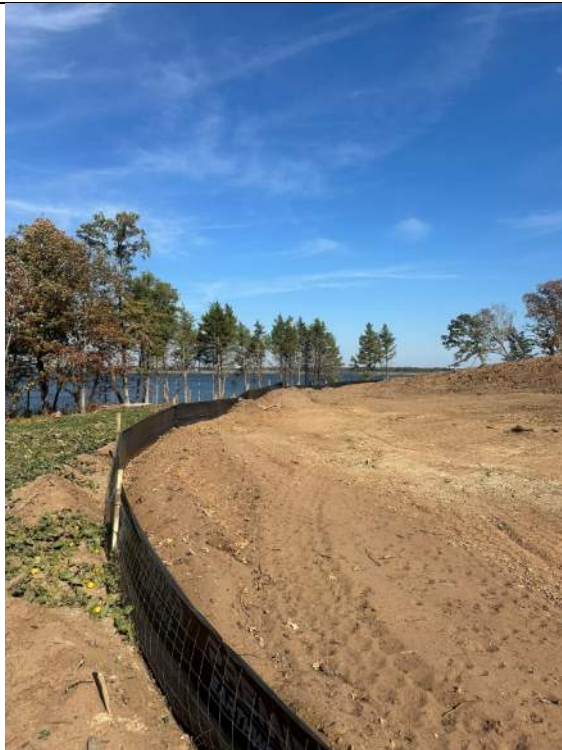
Photo 8: Sediment at 50% capacity of the developer sediment control fencing.
