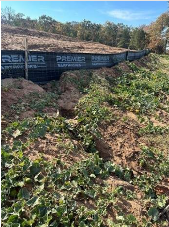
Photo 4: Undercutting of the developer's sediment control fencing and rill erosion.
