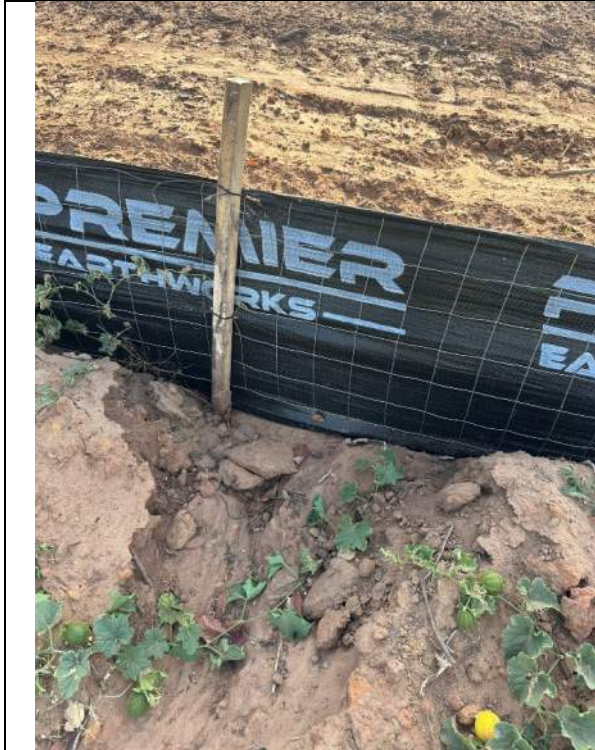
Photo 9: Sediment undercutting developer sediment control fencing.
