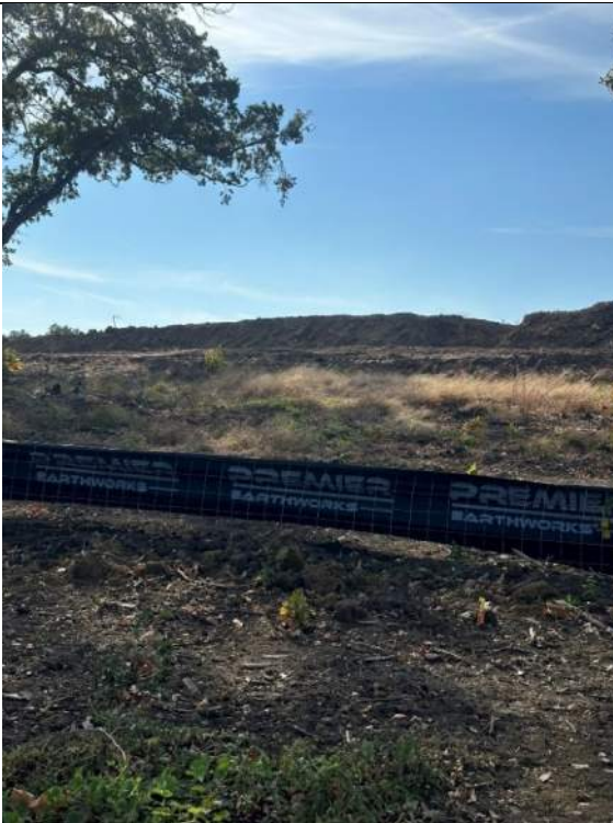
Photo 7: Developer sediment control fencing does not appear to be trenched in.
