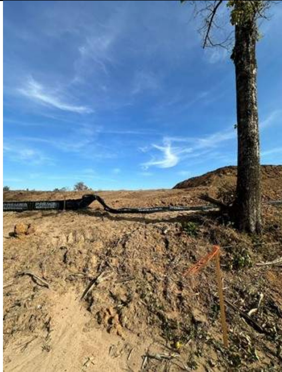
Photo 10: Developer sediment control fencing requiring maintenance.
